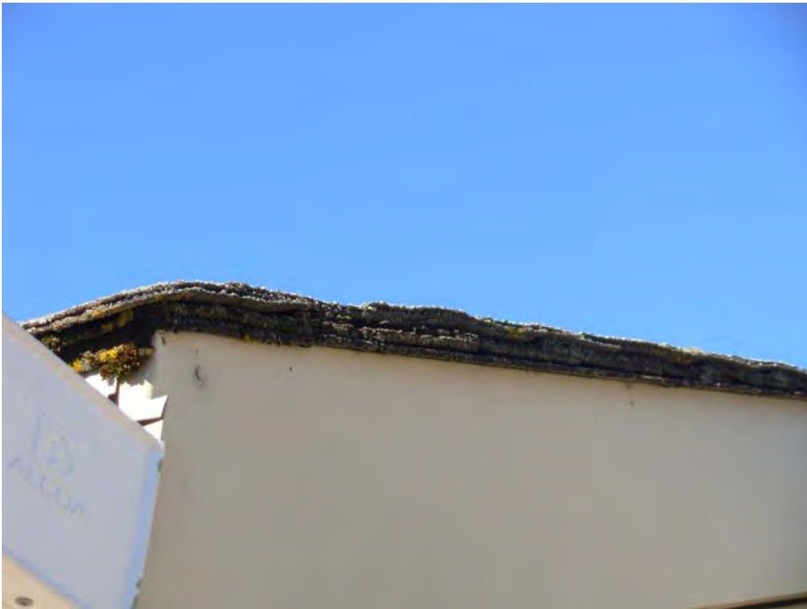
7. Older roofing surfaces appear to be multi-layered
