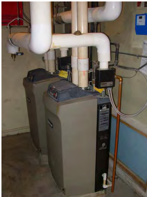
11. Heating boilers, typical at each building
