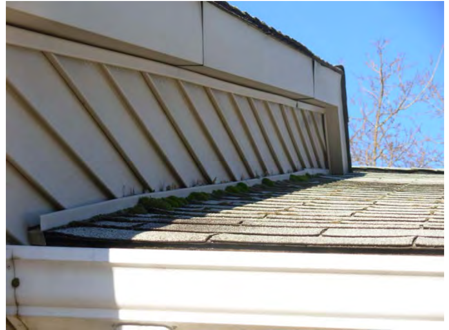
6. Organic material build-up on roofing shingles
