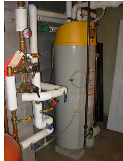
12. Typical DHW tank and mixing valves
