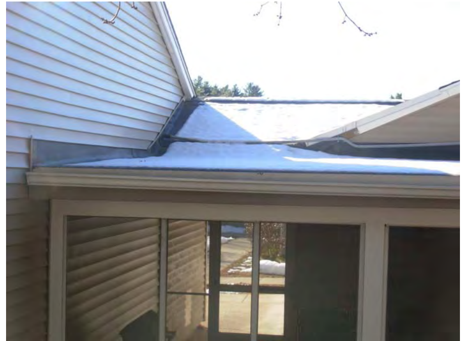
8. Transition porches with flat membrane or rolled asphalt roofing
